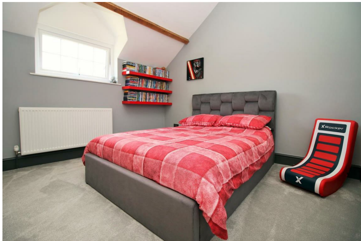
Vaulted beam ceiling. Radiator
